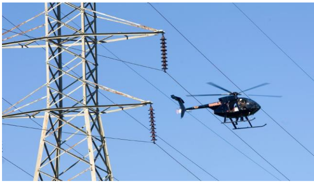
Fig 3:visual inspection by helicopters
